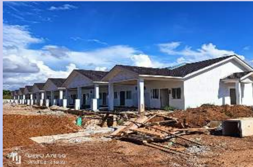
Sanitary wares installation in progress
