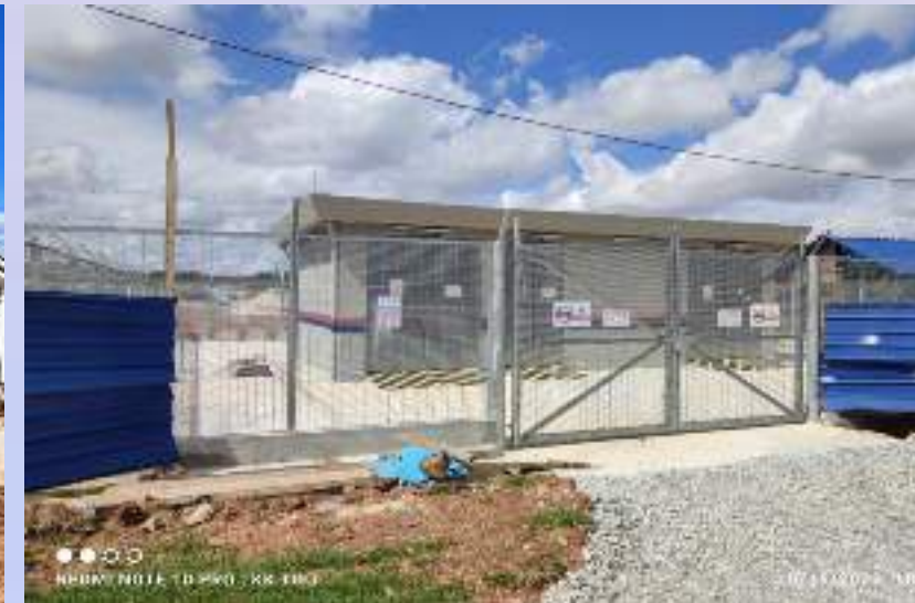
TNB station completed
