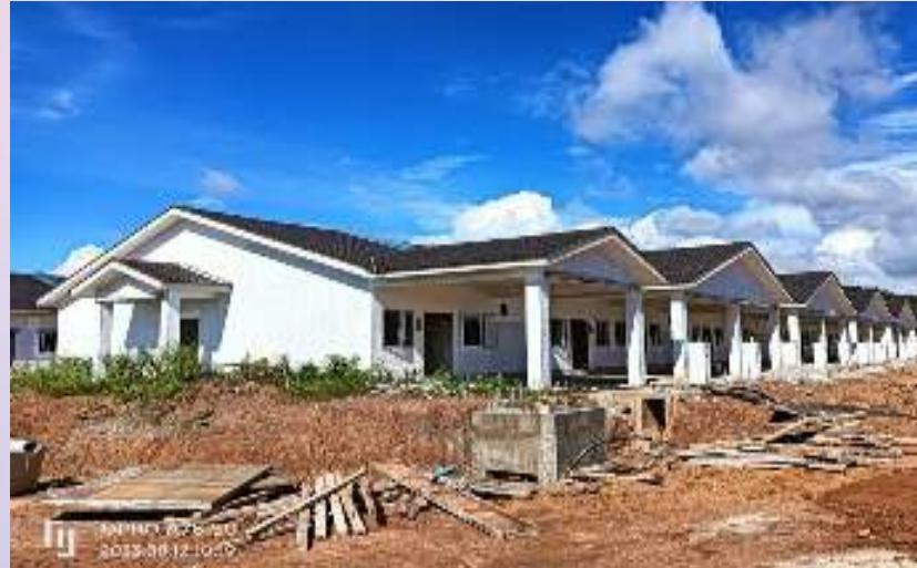
Tiling works completed
