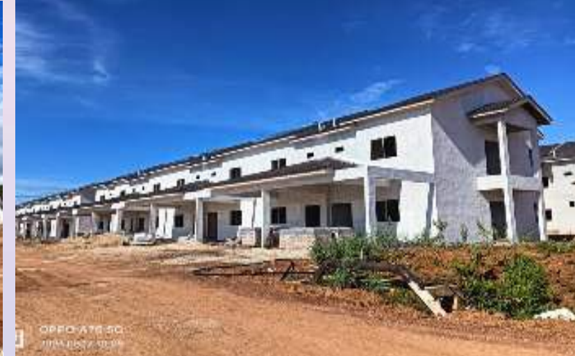
External painting works in progress
