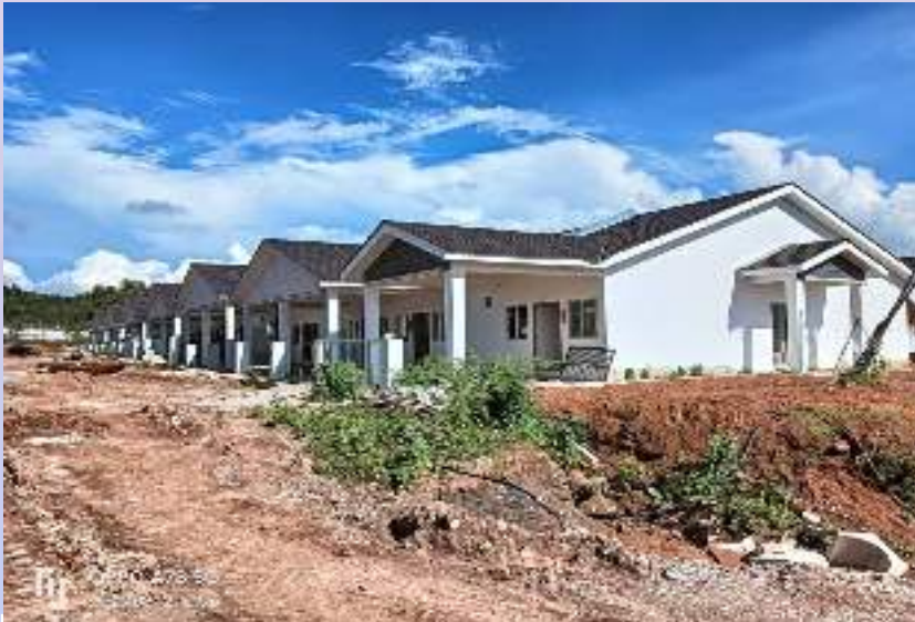
Car porch and apron in progress
