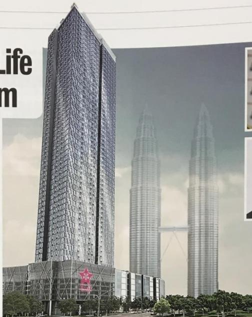
Star Residences, located at the intersection of Jalan Mayang and Jalan Yap Kwan Seng, is Symphony Life's RM3 bil joint-venture development
